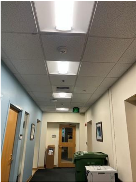
After the upgrade.
