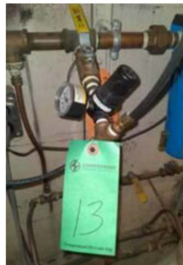
Compressed air leaks identified with green tags on equipment.
