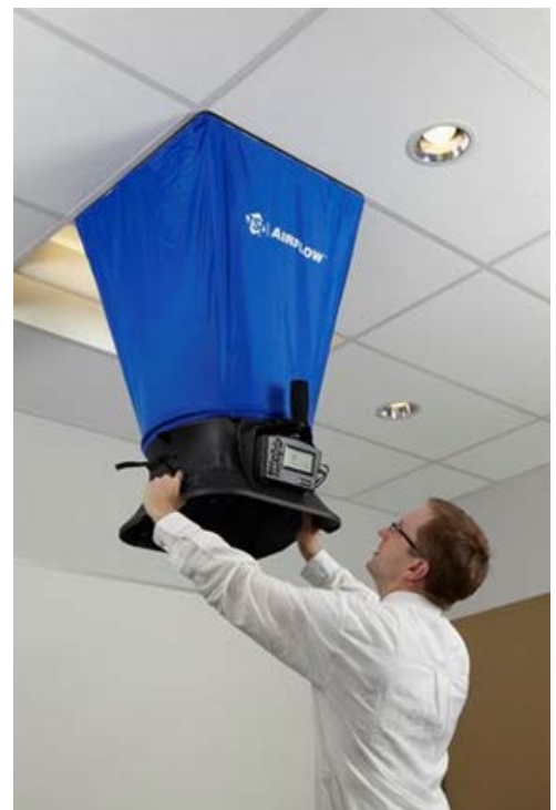
A balometer, or a flow hood, takes supply air readings.
