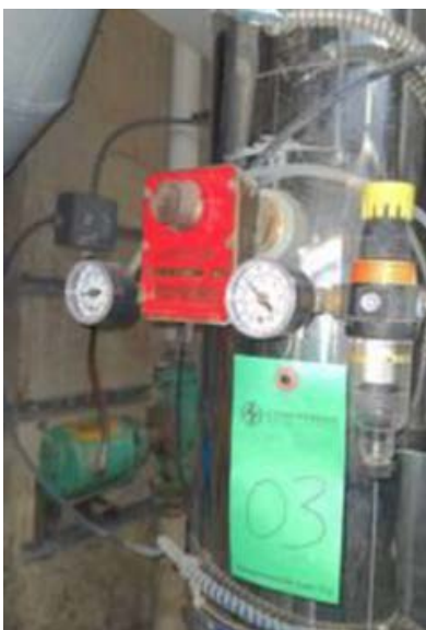
Compressed air leaks identified with green tags on equipment.
