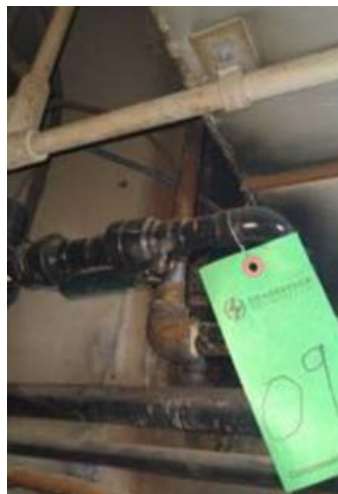
Compressed air leaks identified with green tags on equipment.
