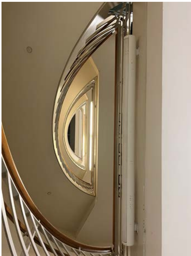
Stairwell from below, before upgrade.
